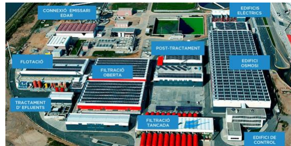
Figure 7. Infrastructure and distribution map of the El Prat de Llobregat desalination plant. Note. The visual identifies the main treatment and supply areas connected to the Ter-Llobregat water network. [17]
