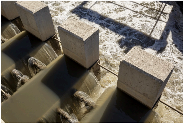
Figure 21: One of the first processes to which water is subjected, the filtration of large bodies through physical barriers.
