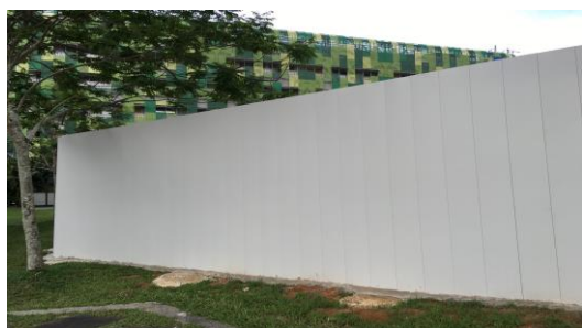
Figure 37. Cemented gap between barriers and ground
