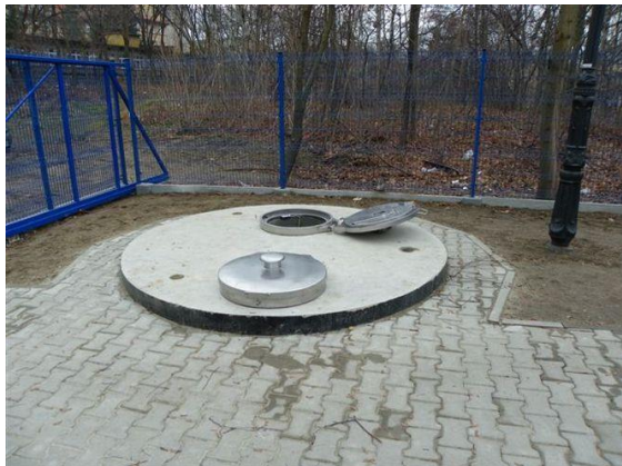
Fig. 1: Water intake in Tęczowa Street.
