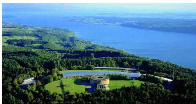
Figure 10: Aerial view of the water treatment plant in Sipplingen on top of a mountain (Sipplinger Berg). Lake Constance with the water intake is on the right side.
